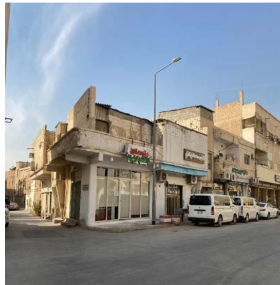
Residential street in the Northern part of the site
