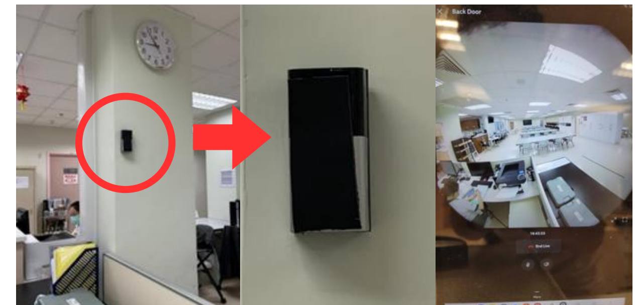
Doorbell Camera System
